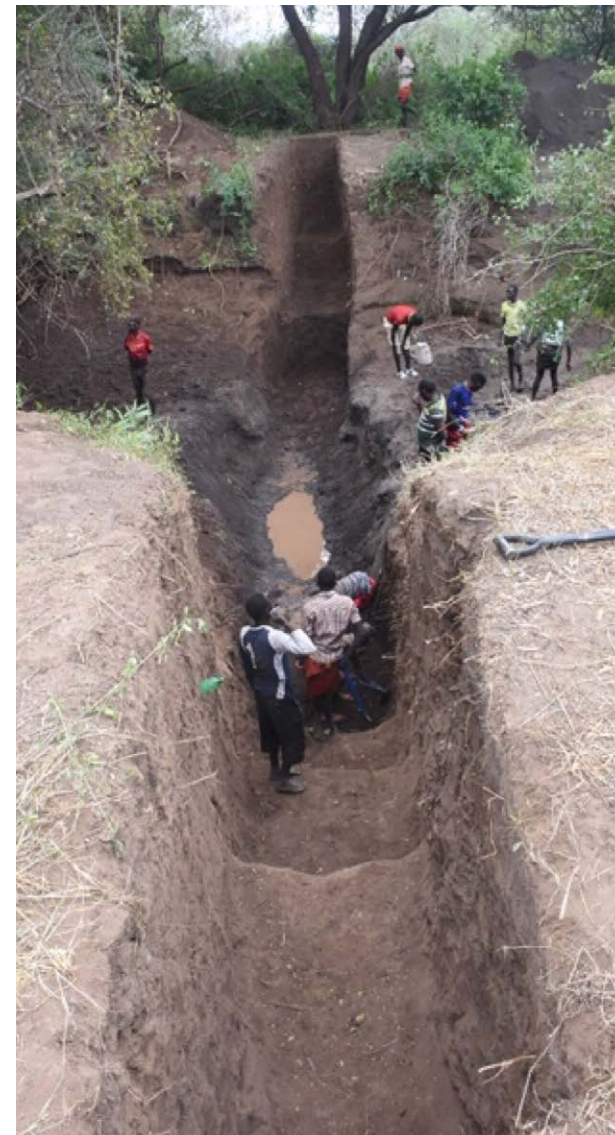
Hand dug trench for installation of concrete sand dam wall
